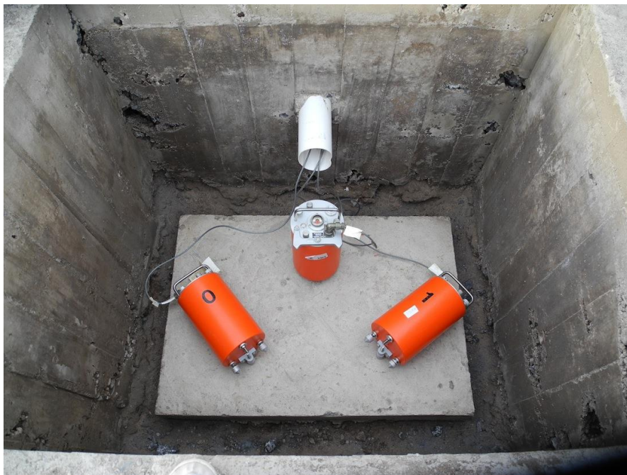
Figure 3. Sensors and vault at Los Leones station (PUMA).
